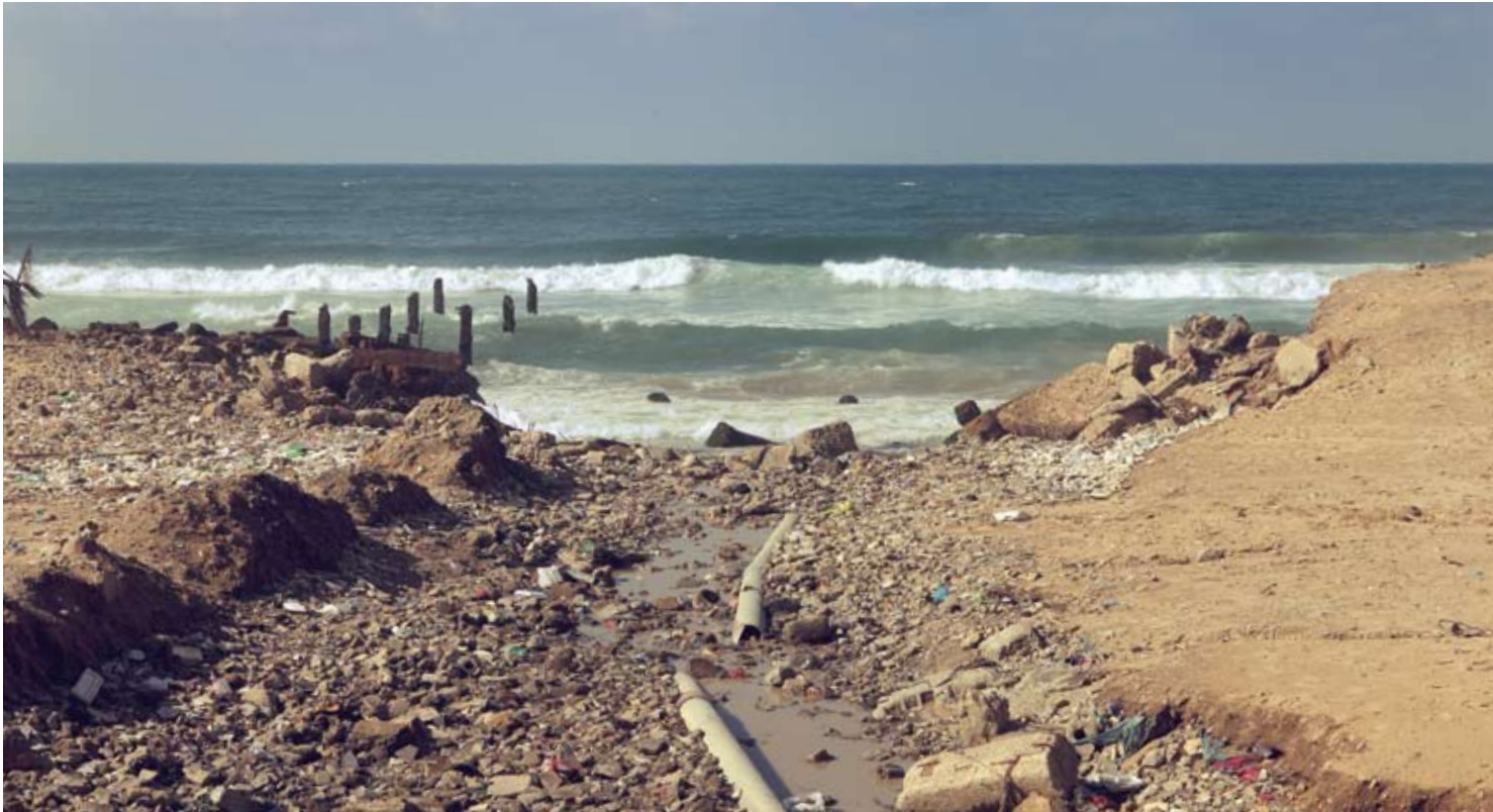
> Sewage flowing into the sea in Gaza. Photo: Anne Paq, activestills.org , 2 February 2012
