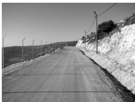
A barrier system under construction around the Ma'aleh Levona settlement, far from its houses, January 2008. The system now includes a barbed-wire fence with an electronic-warning mechanism, a patrol road, and illumination devices.
